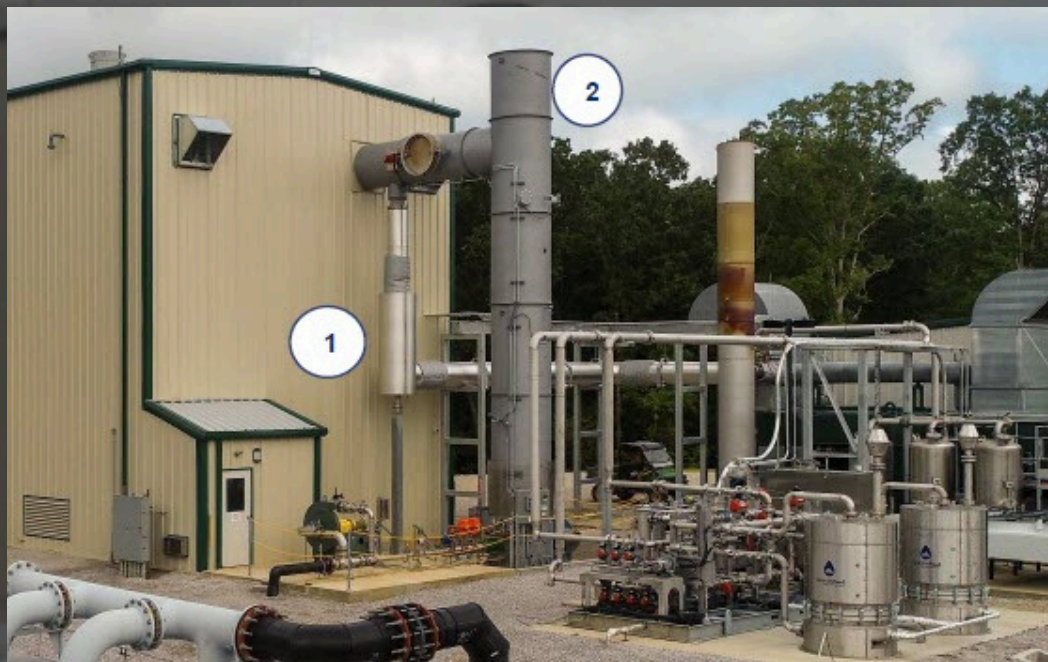
Figure 2. Hybrid configuration showing (1) integration to engine exhaust and (2) landfill gas flare
