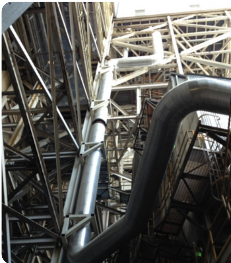
Figure 2. Flue gas ductwork from Bowen's Unit 3 feeding the Heartland Concentrator
